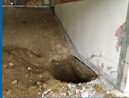
Exposing Existing Footing for New Elevator Pit/Shaft Footing
