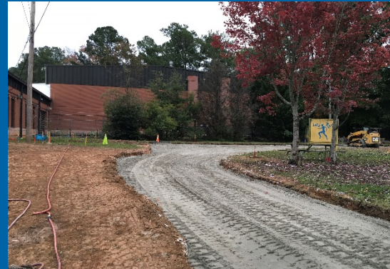
Installation of Gravel Service Road
